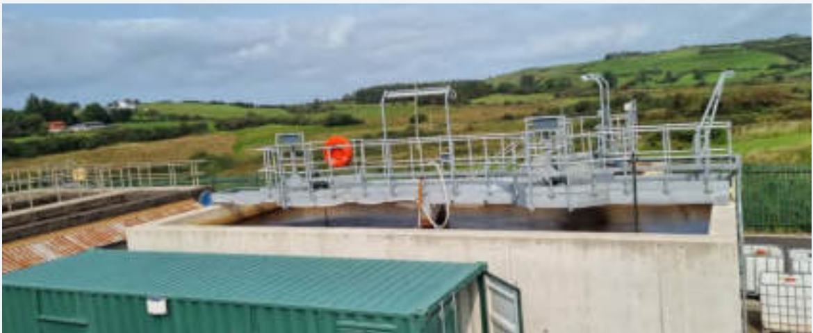
Part of West Clare Water Treatment plant
