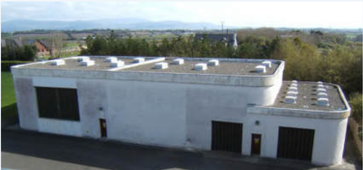
Cavanhill WTP (Chemicals building)
