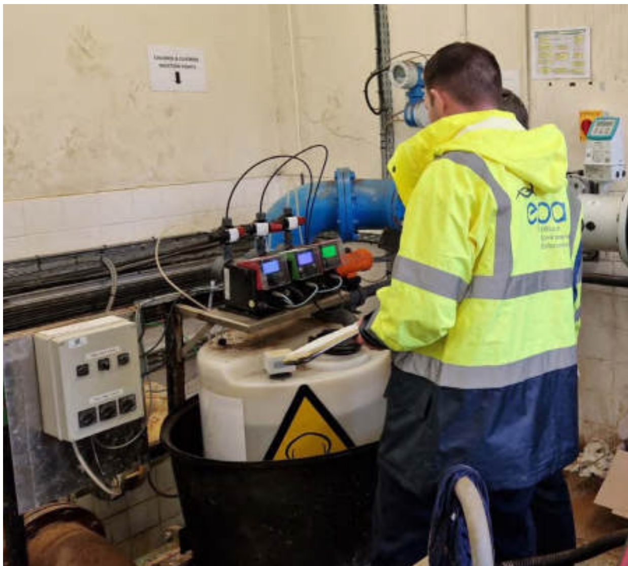
Figure 4.4: Inspection of water treatment plant dosing equipment
