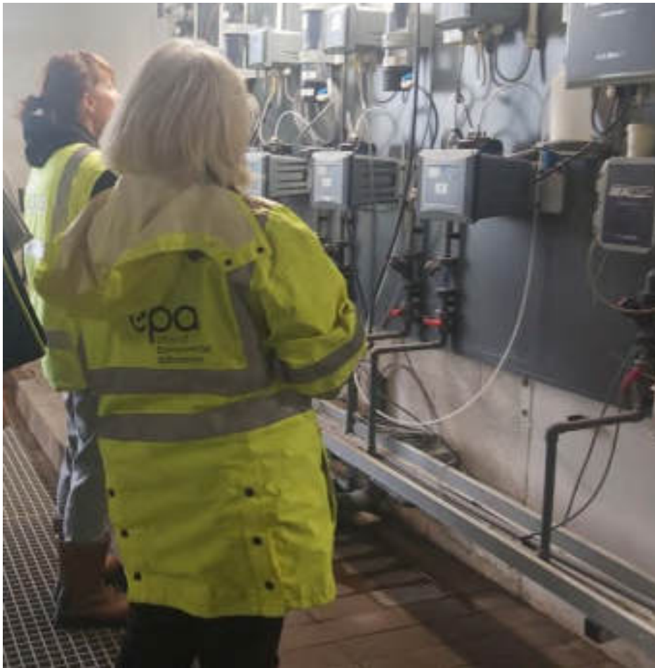
Figure 3.2: Water treatment plan inspection
