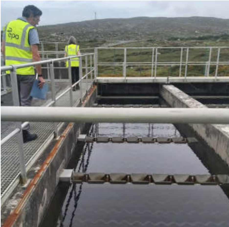
Figure 3.10: Water clarification - solids settle and clear water runs out in the channels
