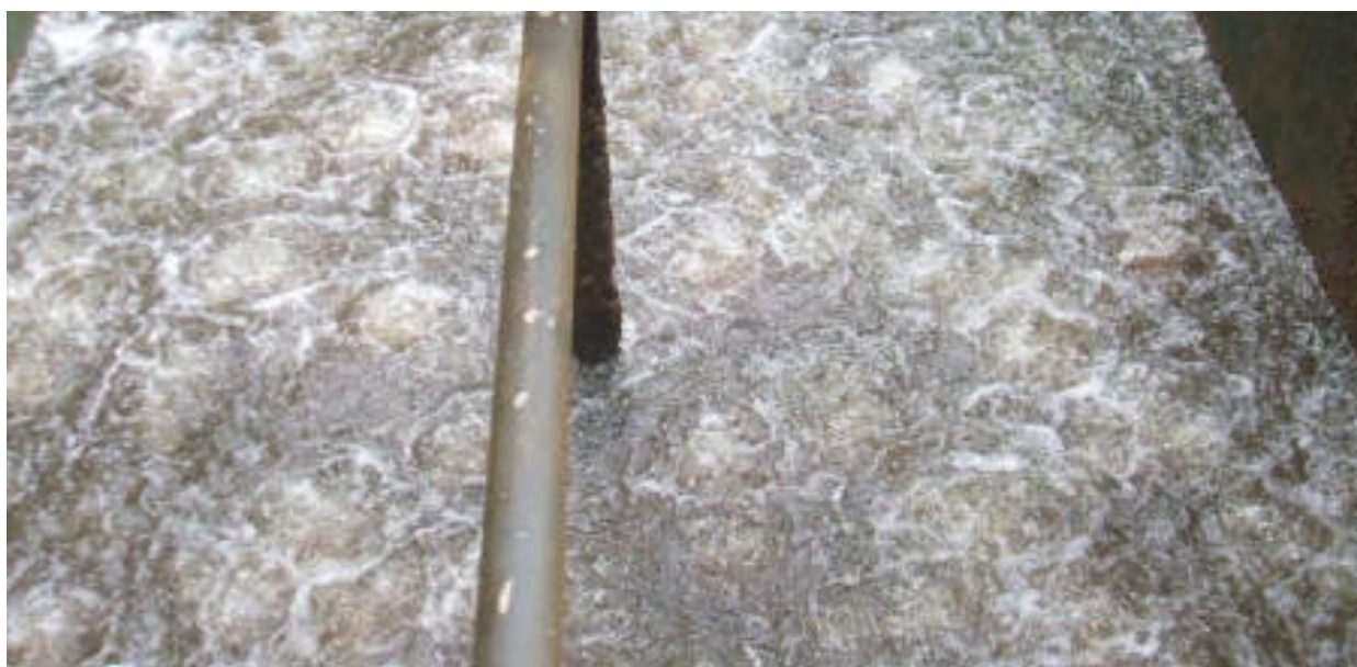
Figure 3.4: Inspecting a water filter (uneven distribution of bubbles means there is a problem with this filter).
